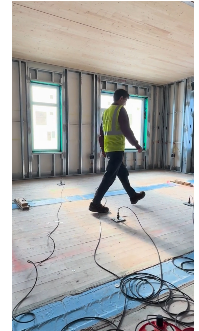
image from Omer Tigli, LinkedIn, floor vibration testing in situ
